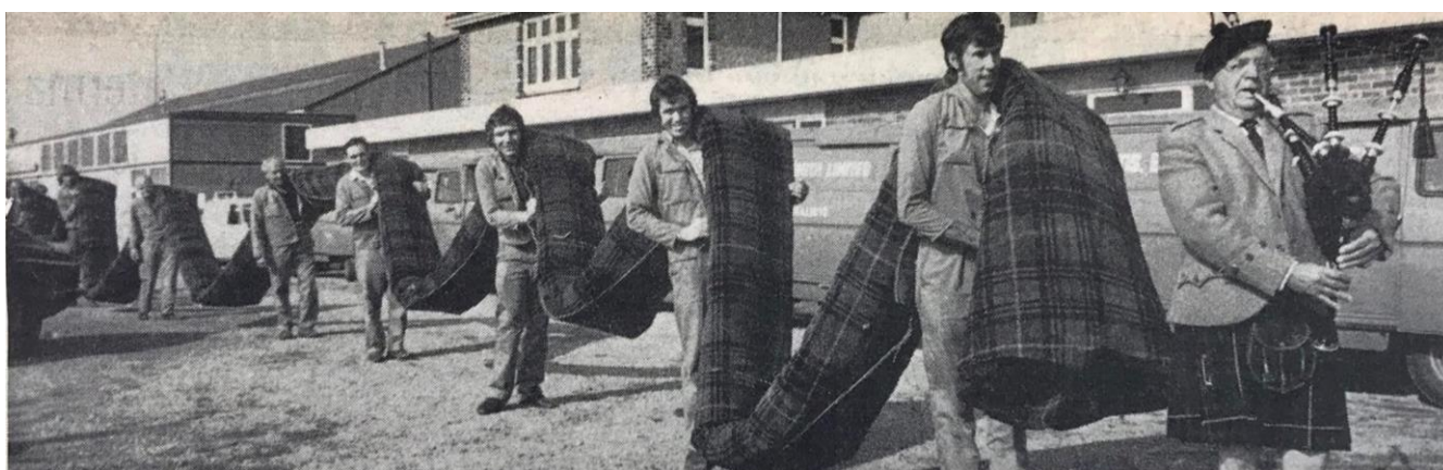
Figure 29 – Piping in the carpet September 1973
